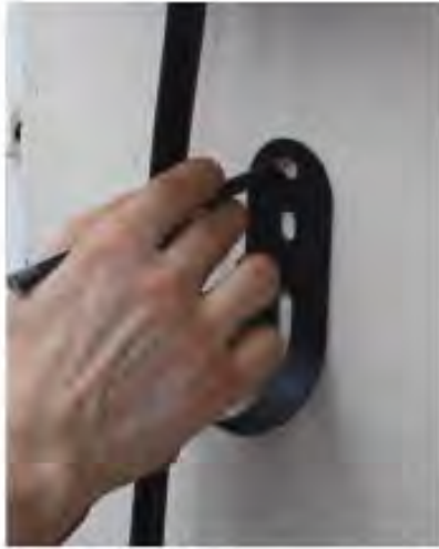
1. Use a pencil to draw location where the hook needs to be punched
