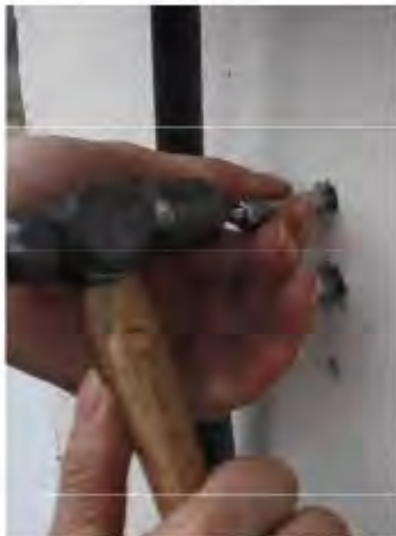
11. Drive the expansion screw in with a hammer
